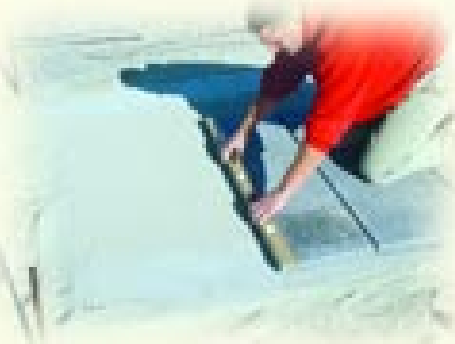
Checking for straight lines
